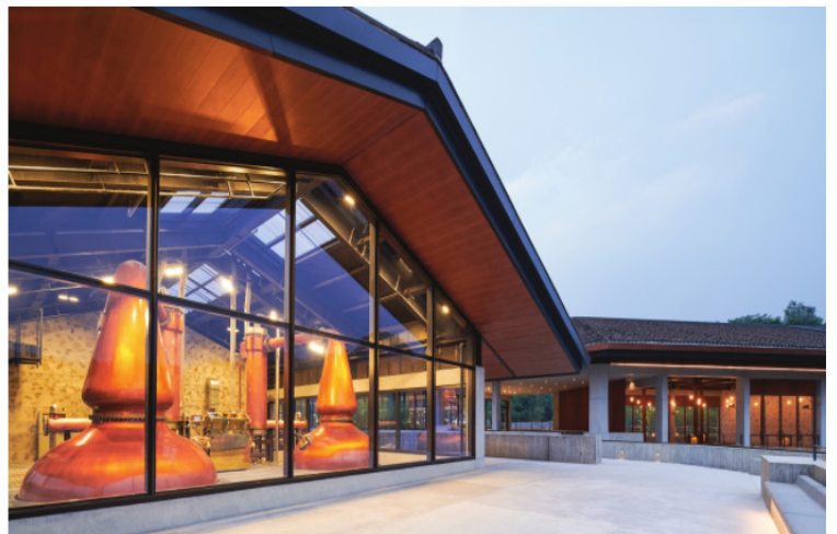
The distillation building of THE CHUAN Malt Whisky Distillery in Emeishan, Sichuan Province photo: courtesy of Pernod Ricard
